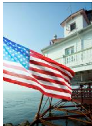
Thomas Point Shoal Lighthouse on Chesapeake Bay proudly displays new JELD-WEN® Windows & Doors.
